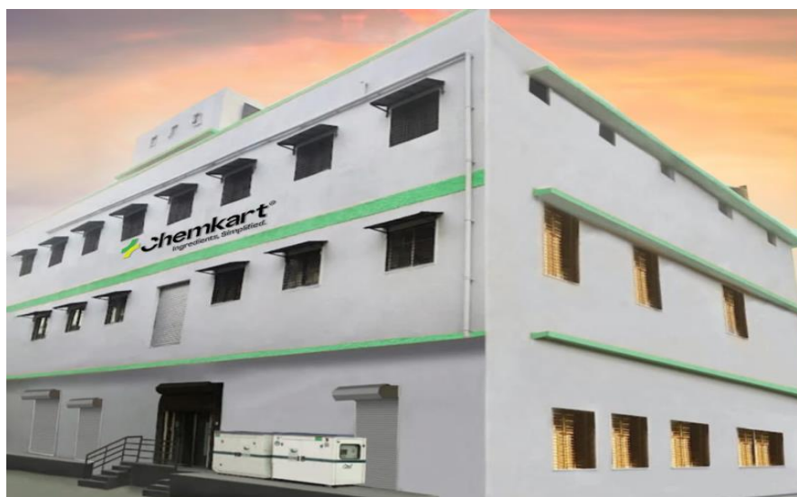
Full Image of Warehouse
