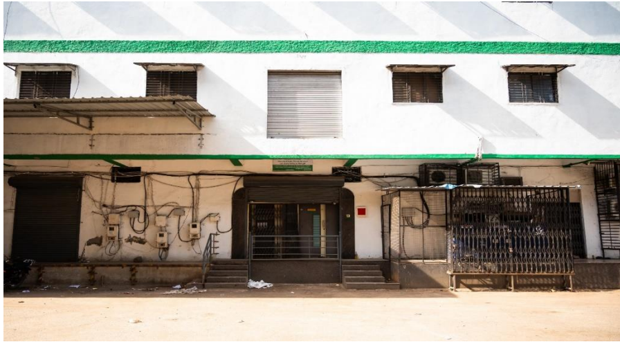
Outer view of the warehouse facility
